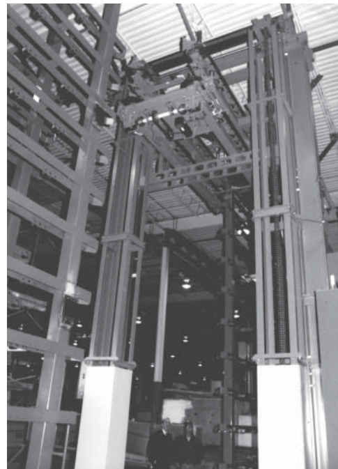
ASRS being set up in the plant. This handles sand cores for a buffer system for casting.
