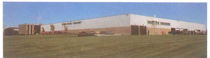
Webb-Stiles Company, main plant and corporate offices in Valley City, Ohio.
